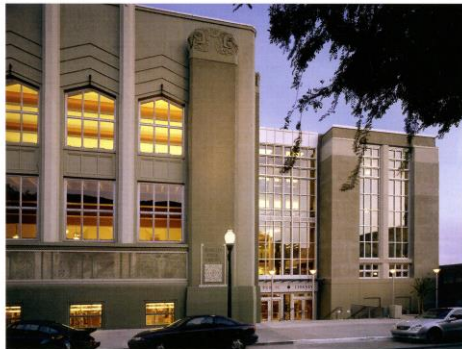
Figure 1. The addition to the right with its connecting hyphen is compatible with the Collegiate Gothic-style library. The addition is set back from the front of the library and uses the same materials and a simplified design that references, but does not copy, the historic building. Photo: David Wakely Photography.
